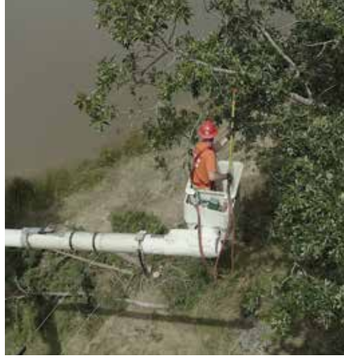
Right-of-way maintenance crews trim vegetation away from power lines on an updated eight-year cycle. This helps keep members connected.
