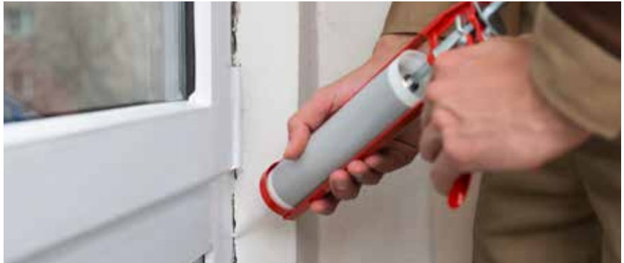
Weatherstripping and caulking around doors and windows is a cost effective way to seal up your home this winter. It will help keep chilly air outside and heated air inside.
